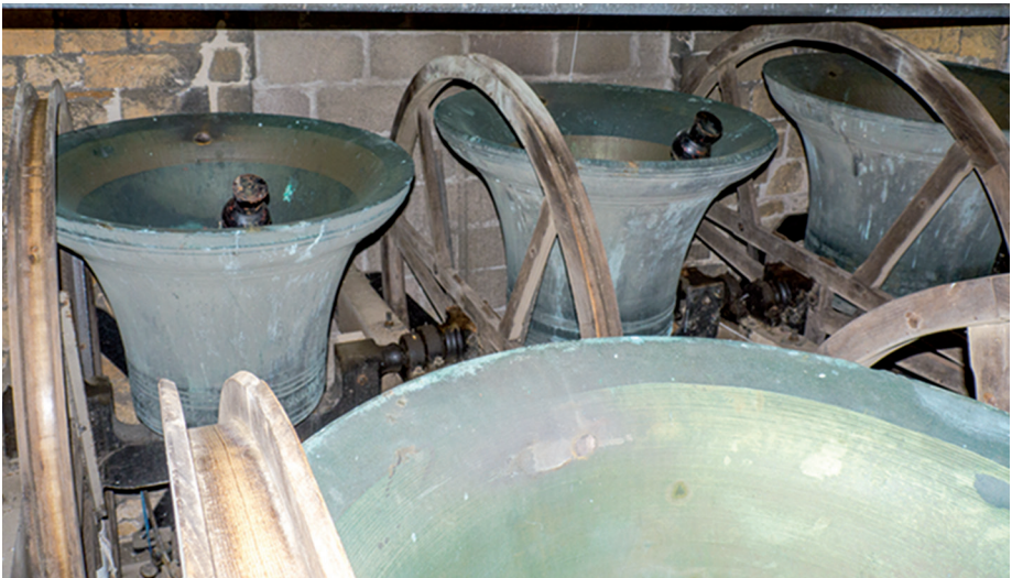
At the rear left, is the No. 4 bell, the oldest in the tower; with, to its right, the No. 5 and then the tenor. The bell in the front is No. 3. The bells are raised, i.e. mouth up, ready for ringing.
